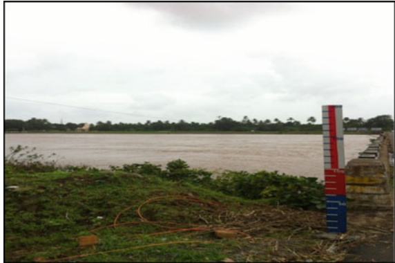
Fig. 6 Flood level indicator
